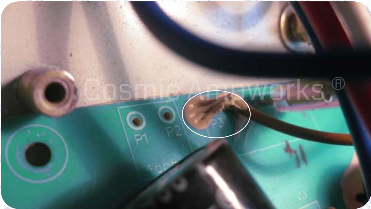
Figure 27. Negative feedback for the presence control (running to the center wiper of the 1M NFB potmeter; Figure 12) is taken from point P3, connected to the 8 Ohm output transformer speaker tap. P3 may be covered in some insulating substance from the factory – if it's difficult to remove, just solder the wire to the trace on underside of the board (which also holds spade connector T14).
